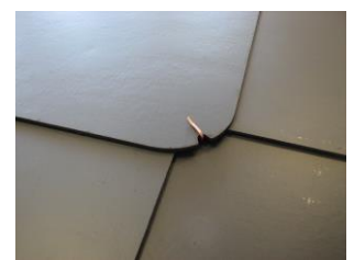
Placing the diamond slate in the drive hook
